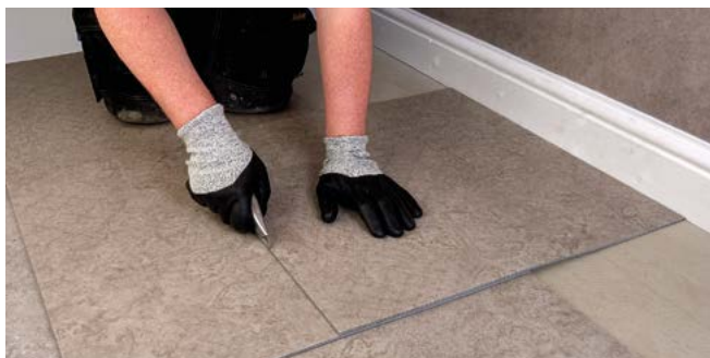
Figure 8 Measuring using an overlapping tile
