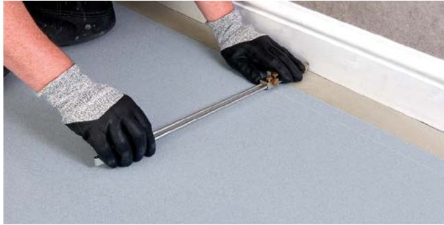
Figure 11 Scribing the wall profile
