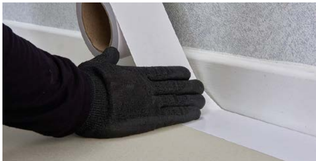
Figure 12 Use double sided Polyflor recommended tape
