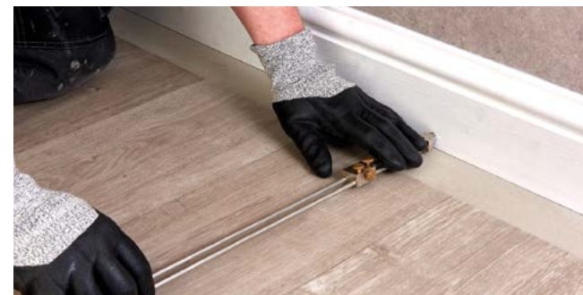
Figure 2 Scribing the wall profile
